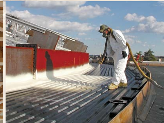
Roof Insulation
