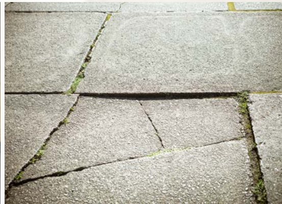
Concrete Lifting
