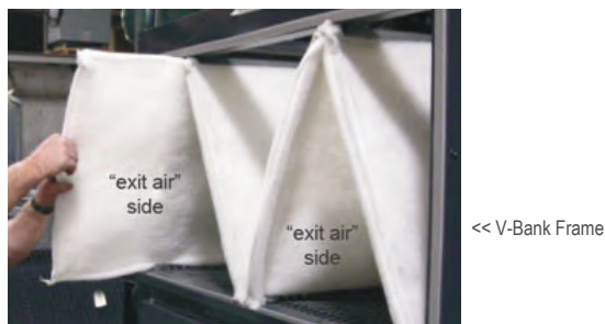
FIGURE 8: Side-Load, Side-Access, Frame-Style Configuration
